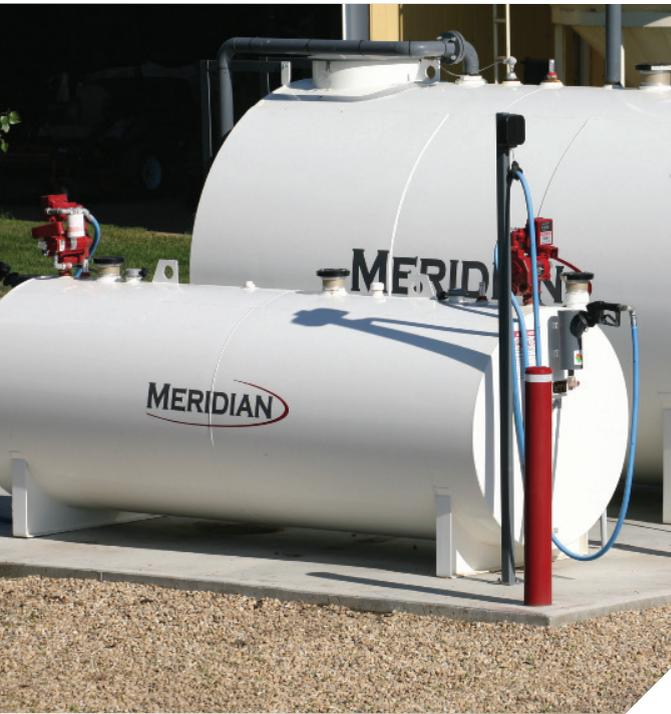
Meridian Double Wall Containment Tanks prevent costly leaks and provide environmentally safe storage.
